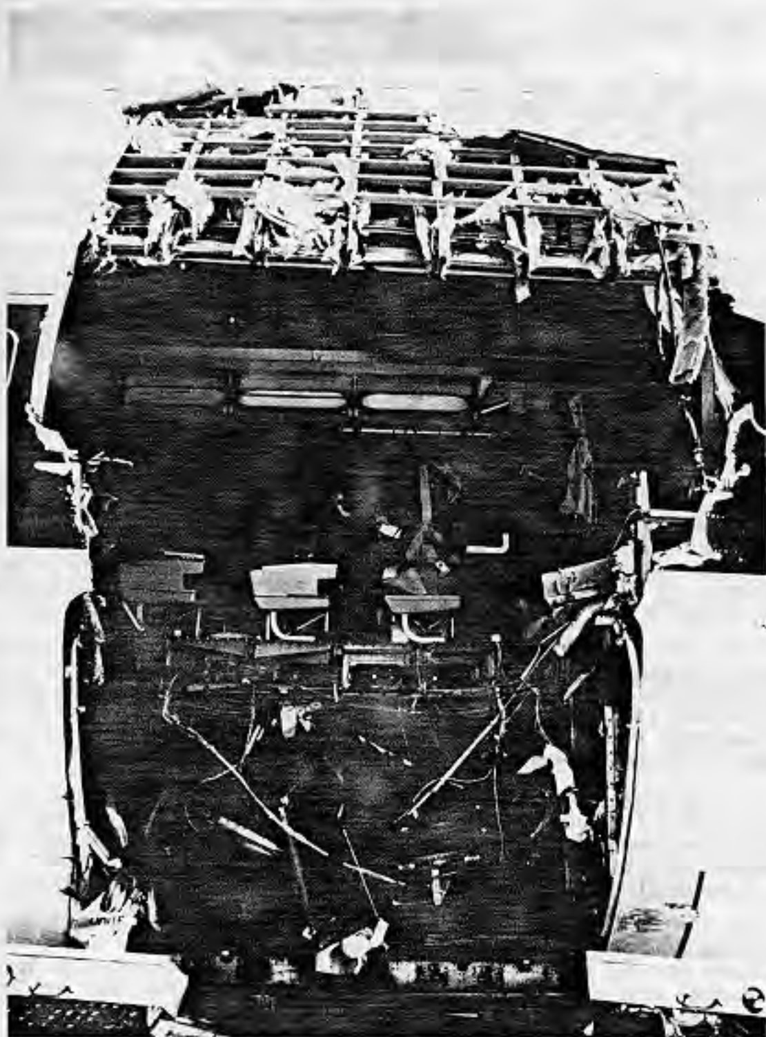
Figure 2.--Close-up view of hole and surrounding structure damage.
